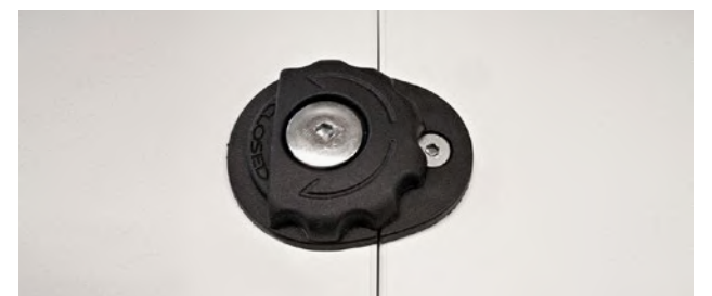
Anchoring by means of plastic clamp e=4mm
