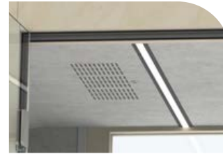
Sensor controlled led lighting.
